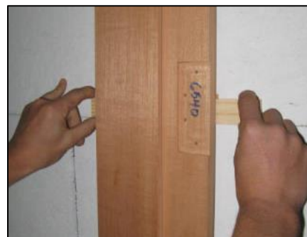
Figure 5 – Shim Placement 2
