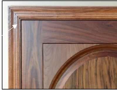
Figure 3 – Checking Door Spacing
